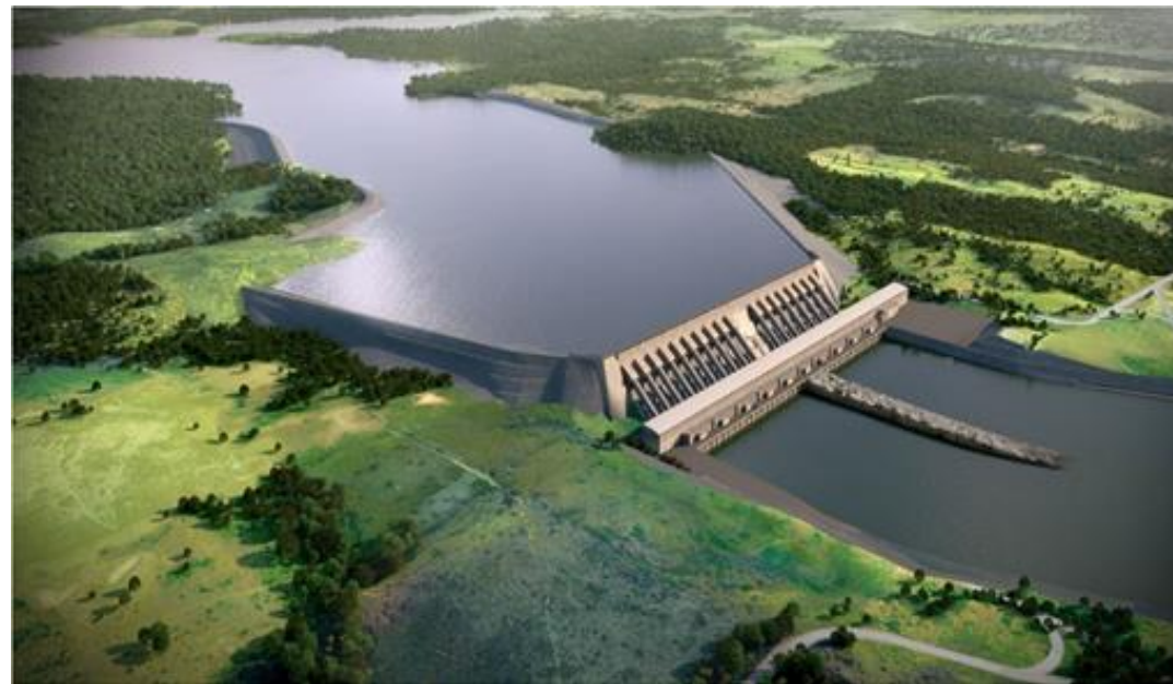
Run-of-river Power Plant
