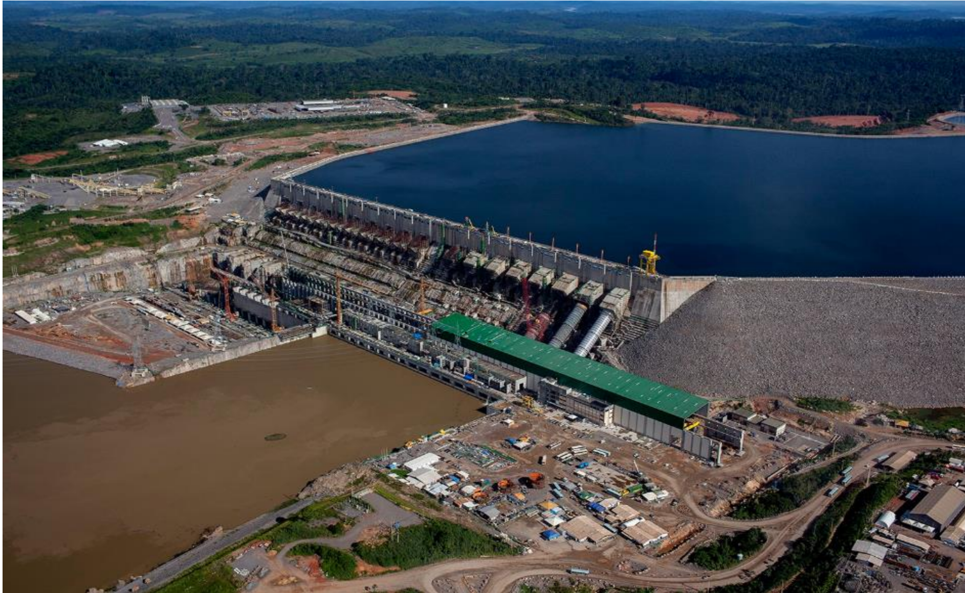
Photo of early construction work - Belo Monte Hydro Power Plant
